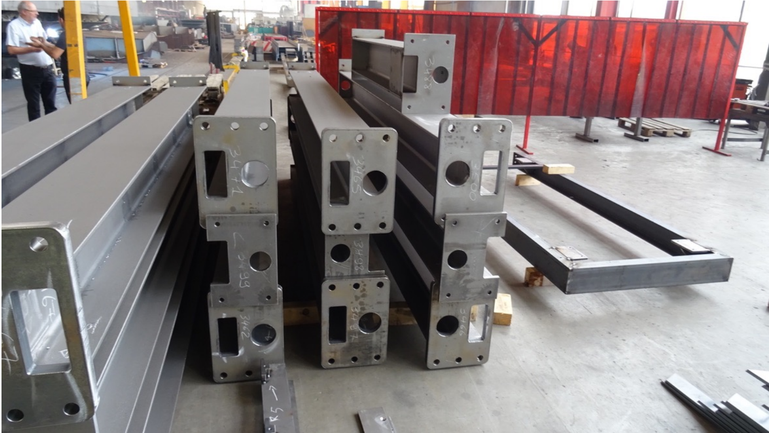
Fabrication, ateliers Sottas SA, photo A. Nussbaumer
